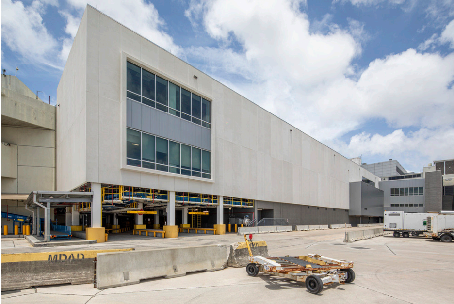
Gurrimatute was part of a team with PDS, Inc. design the New South-Central Checked Baggage Inspection System, Checked Baggage Reconciliation Areas Baggage Handling System Building at Miami International Airport. This 71,000 sf, $177M project achieved LEED Gold Certification and was designed for Sea Level Rise.
