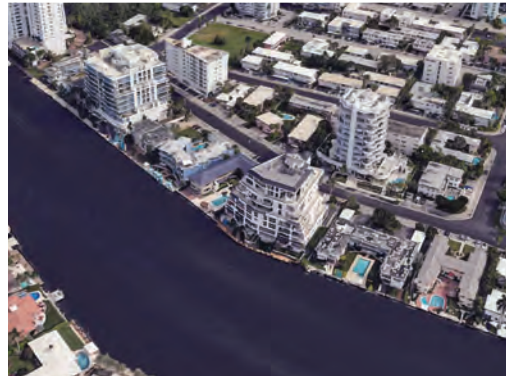
6 - SOUTHWEST CORNER SHOWING NEIGHBORING PROPERTIES
