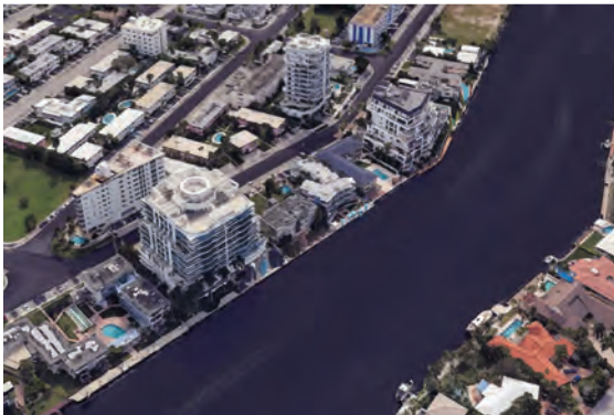
5 - NORTHWEST CORNER SHOWING NEIGHBORING PROPERTIES
