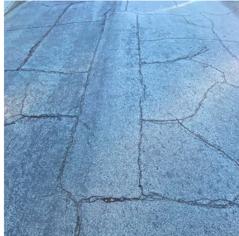
Block Cracking
