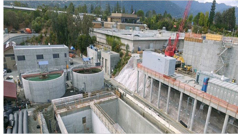
RWTP Reliability Improvements ($720 Million)
