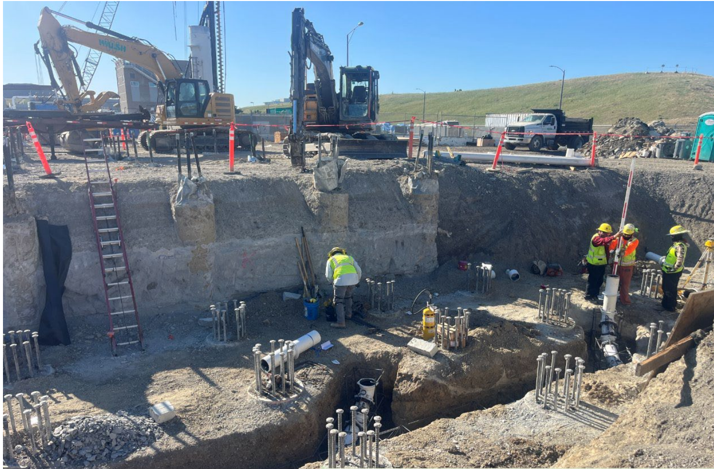
90-ft deep Auger Cast Piles for Thickening & Dewatering Building
