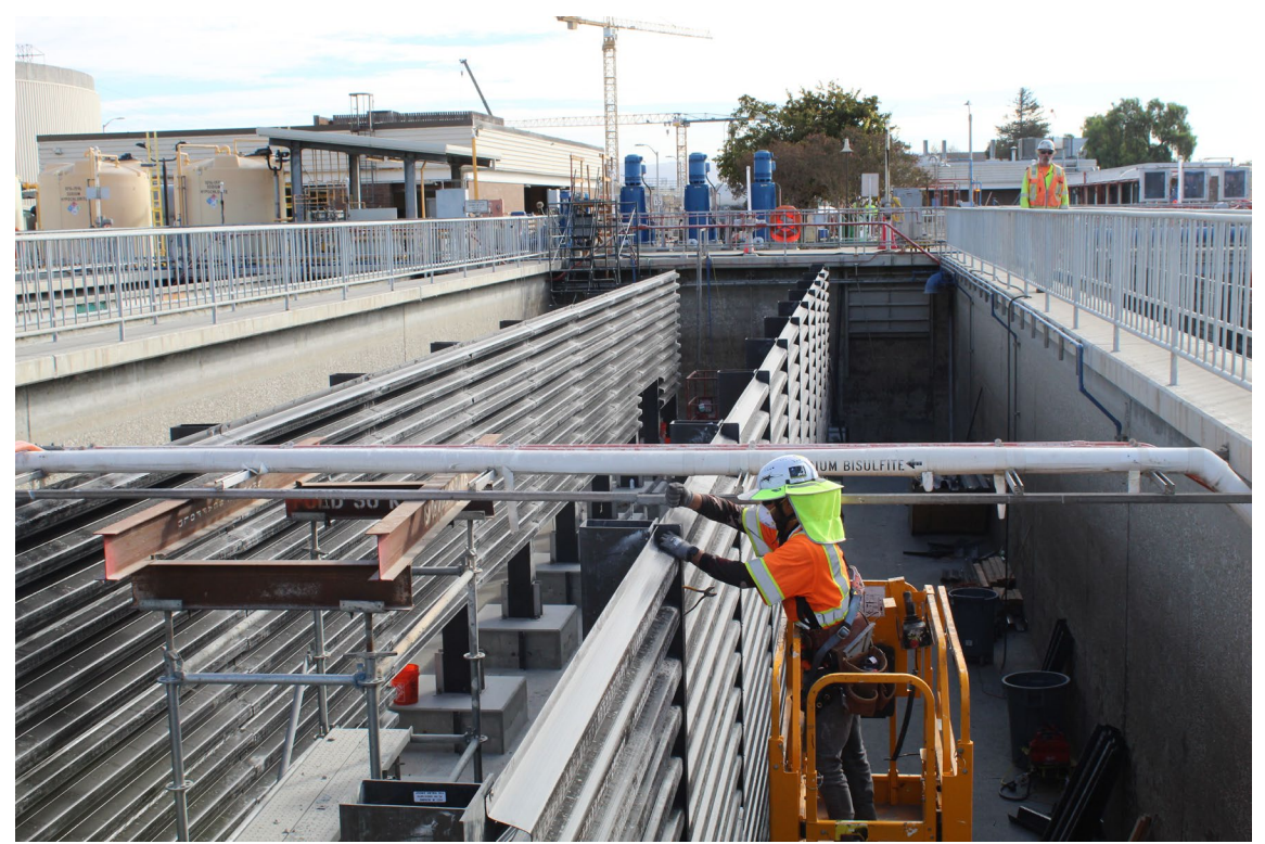
New Baffle Walls in Chlorine Contact Tanks
