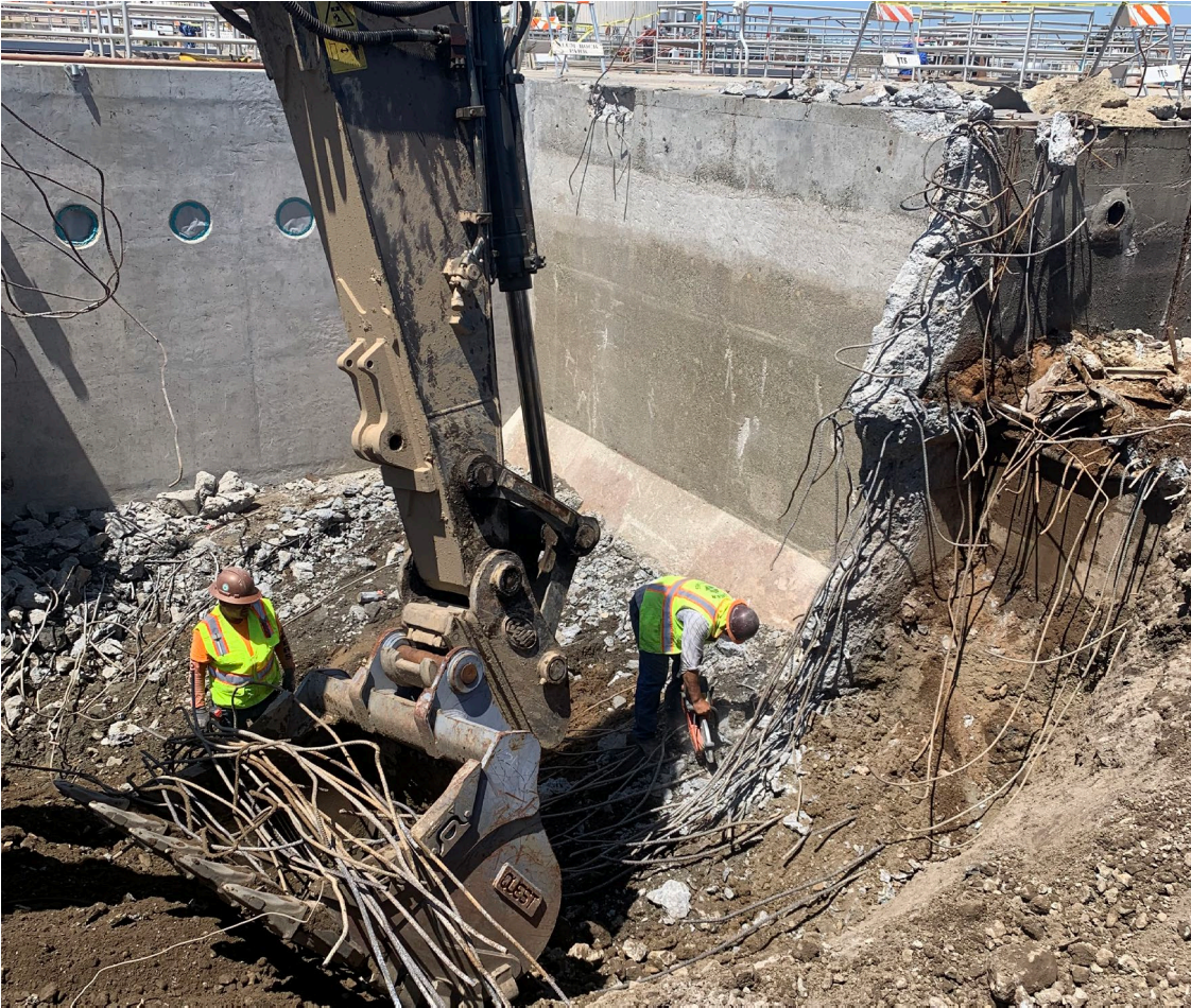
Demolition of Existing Primary Sedimentation Tanks
