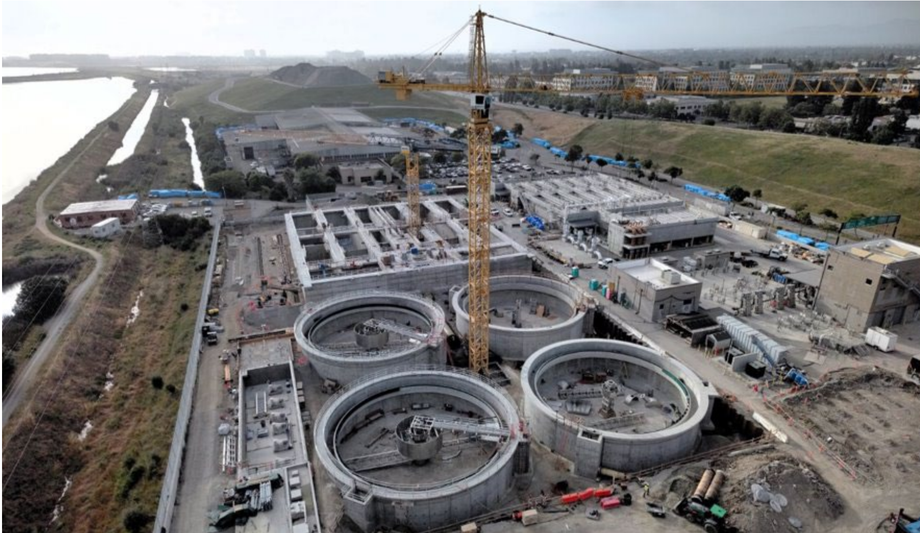
New Secondary Treatment Facilities
