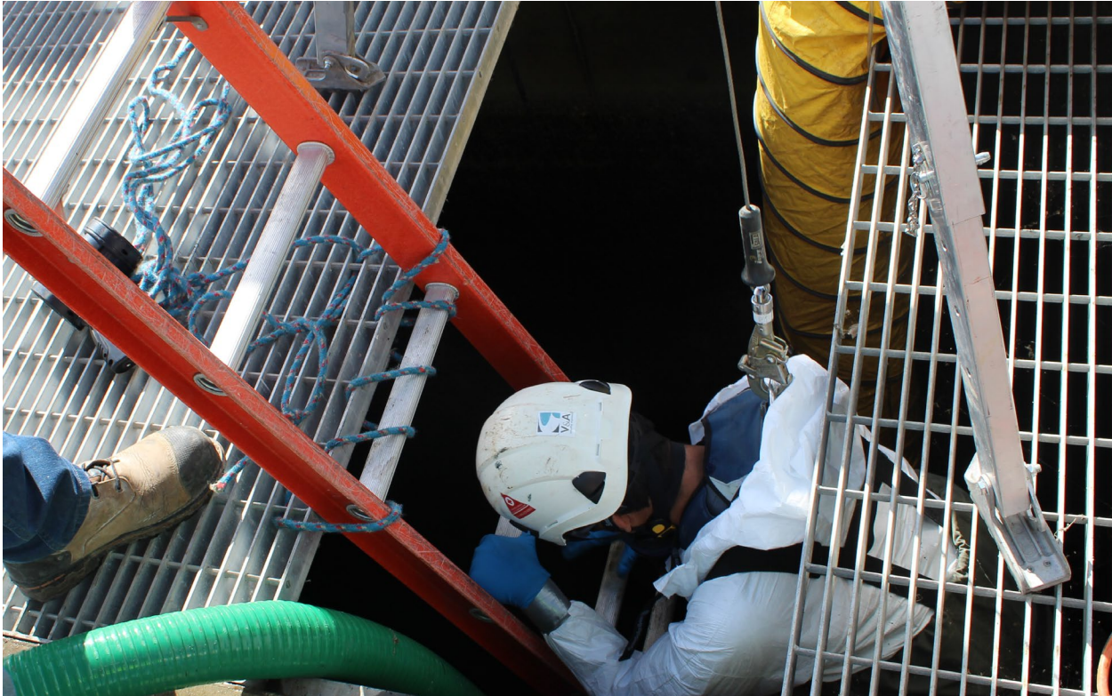
Visual Inspection of Existing Facilities
