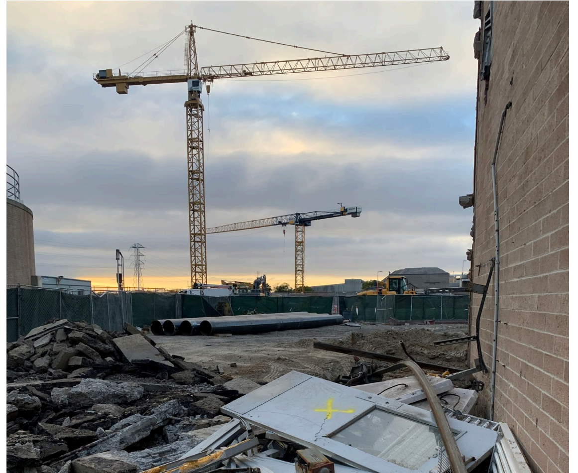
Demolition of Existing Primary Control Building
