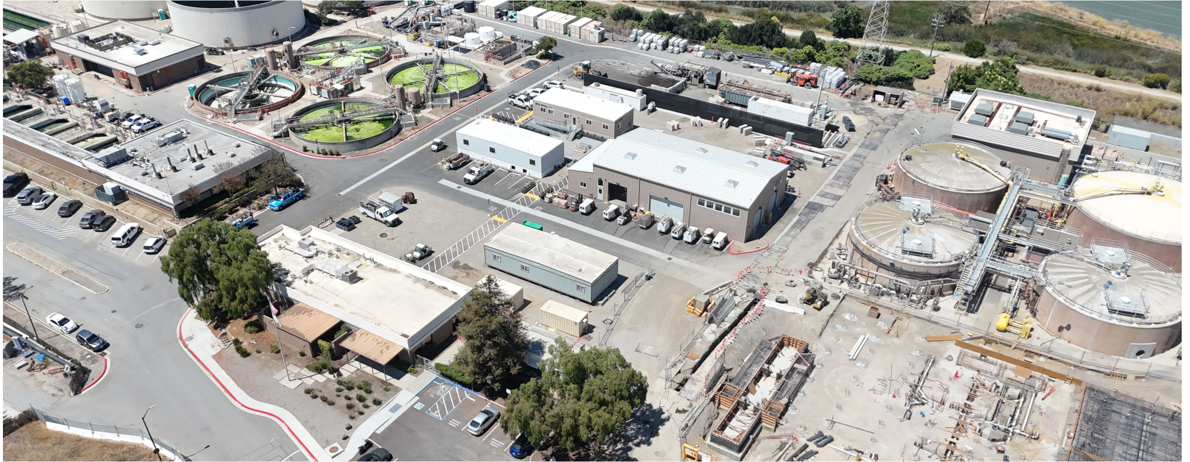
New Temporary Maintenance Shop and Office Trailer Complex
