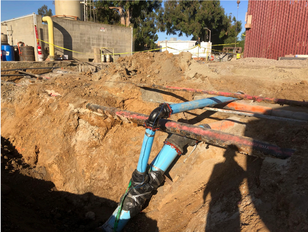
Field Adjustments to Installed Pipelines
