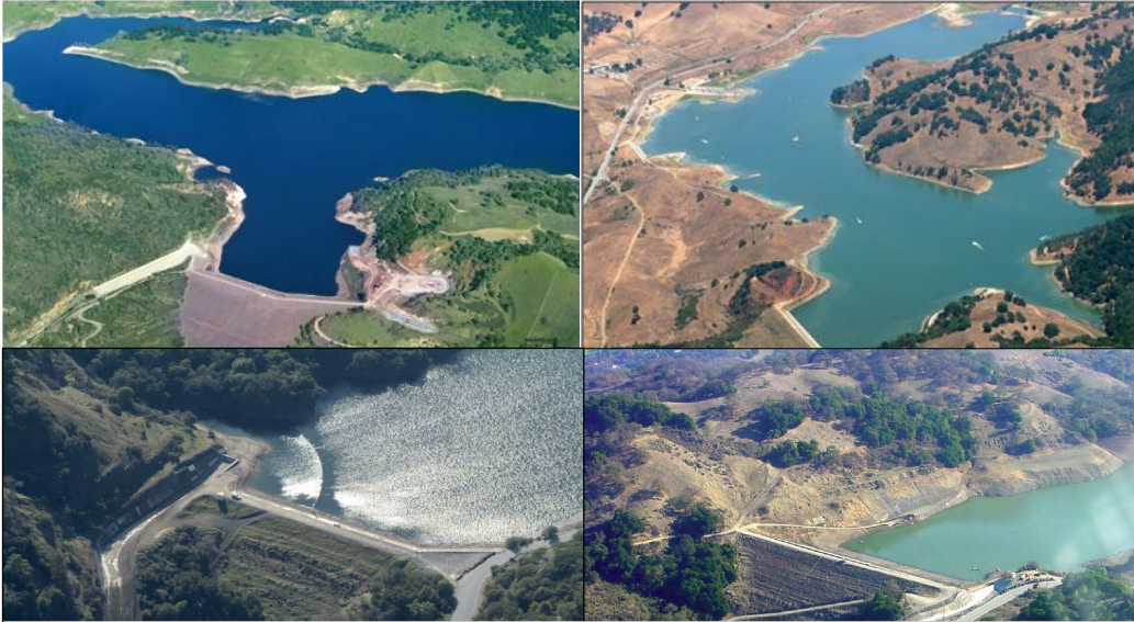
Dam Seismic Retrofits/Improvements ($1,771 Million)
