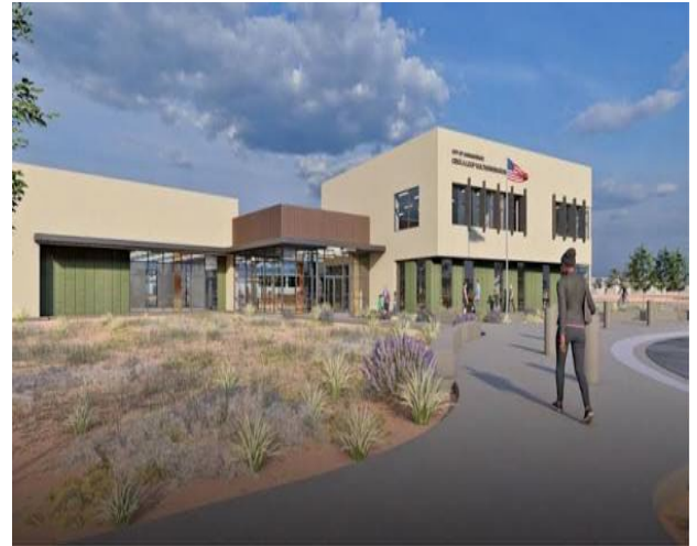
Conway Wood Northwest Multigenerational Center
