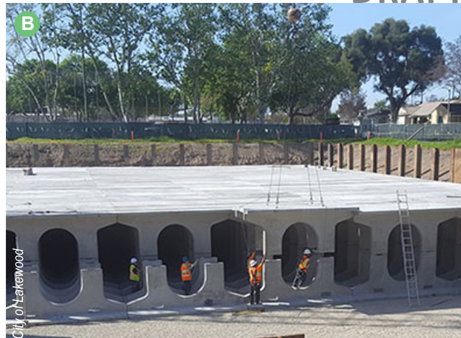
Example of Subsurface Infiltration System at Bolivar Park in Lakewood, California
