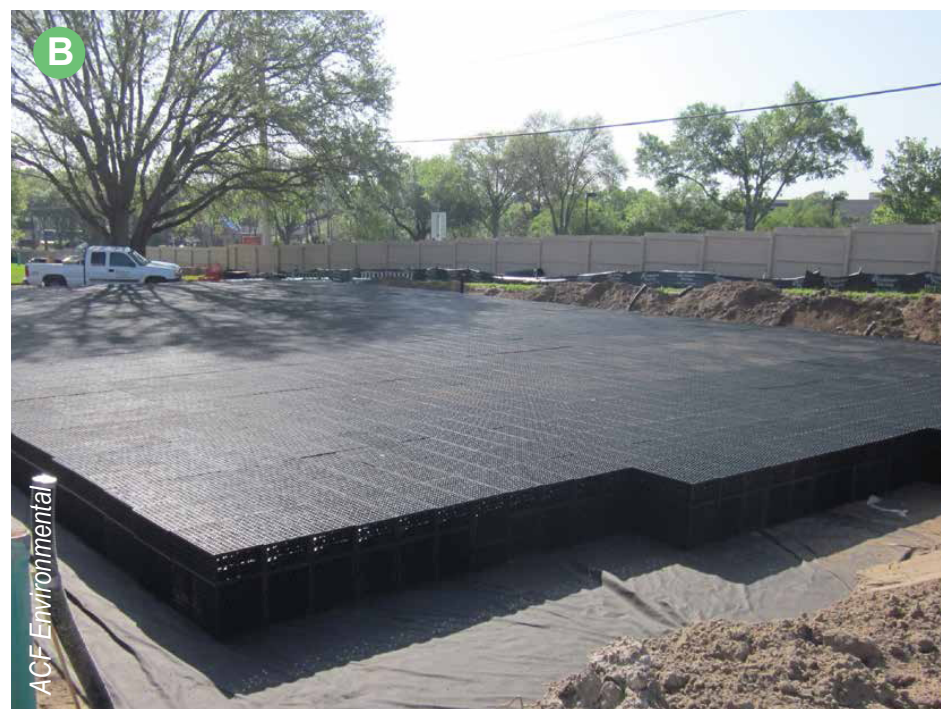
Example of Subsurface Cistern at Patient Towers in Gainesville, FL
