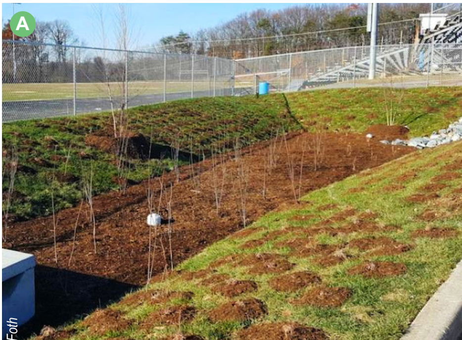
Example of Bioretention System Integrated into Park Setting at High Point High School in Beltsville, Maryland
