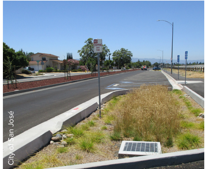
Figure 6-7. Chynoweth Avenue Bioretention
