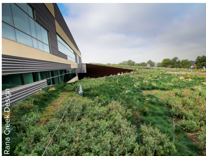
South San José Police Station Green Roof
