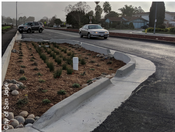
Bioretention Curb Extension on Chynoweth Avenue
