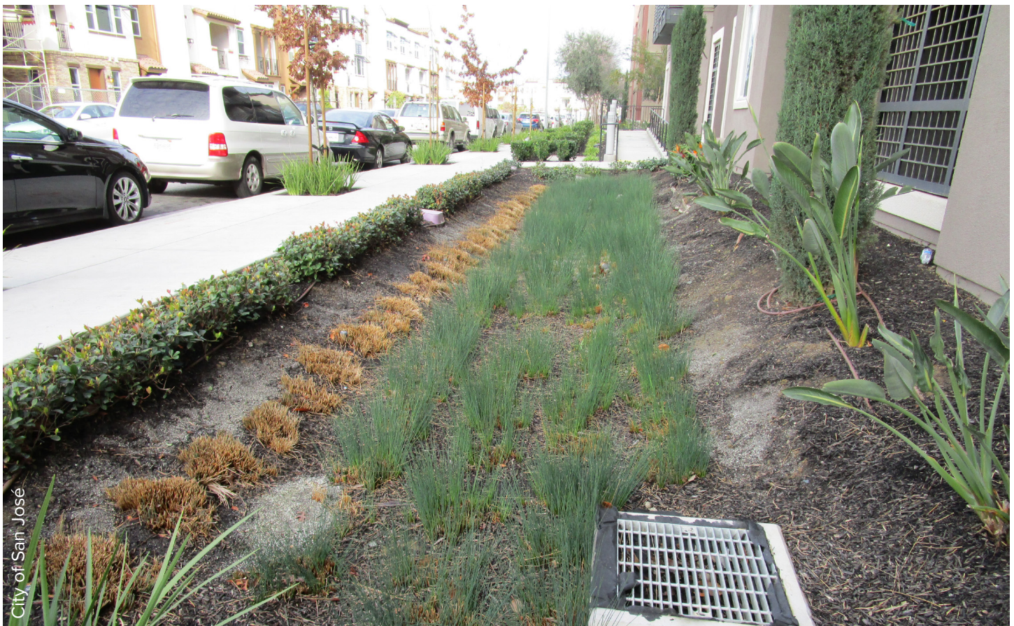
Bioretention at Montecito Vista Urban Village
