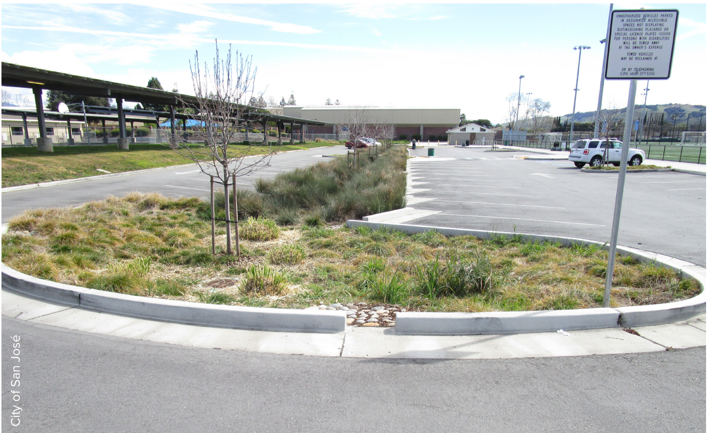
Bioretention in Park Parking Lot
