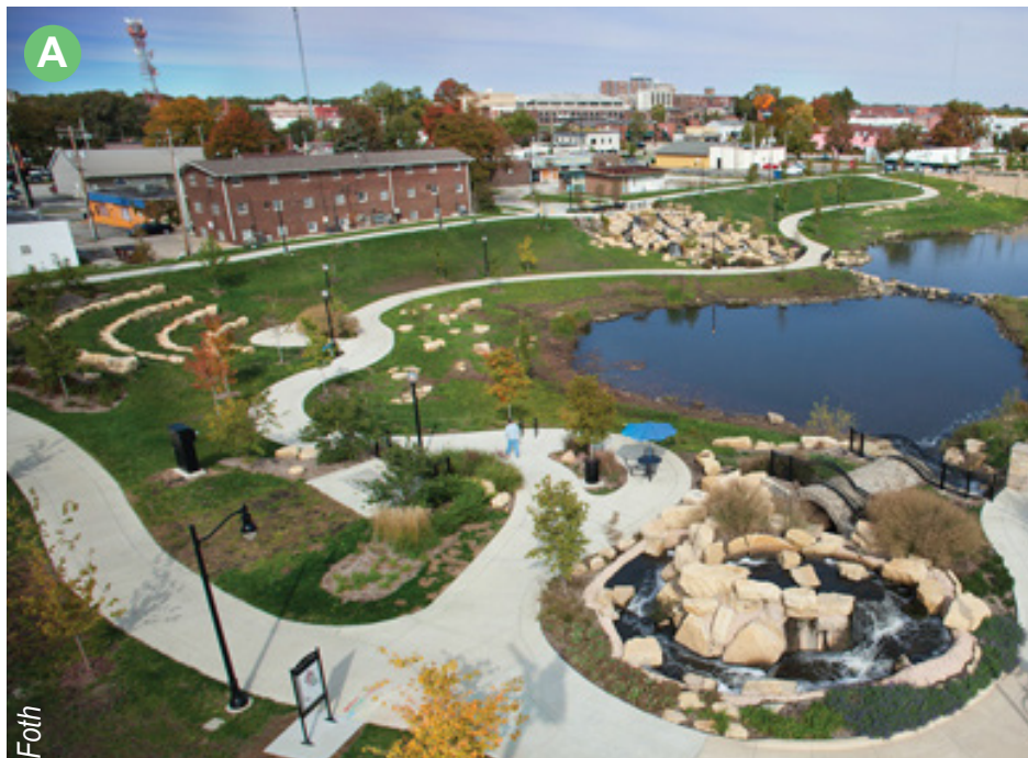
Example of Regional Stormwater Treatment Integrated into Park Setting at Helms Park in Champaign, Illinois
