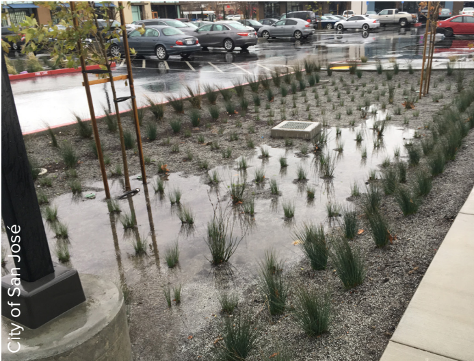
Bioretention at Brokaw Commons in San José
