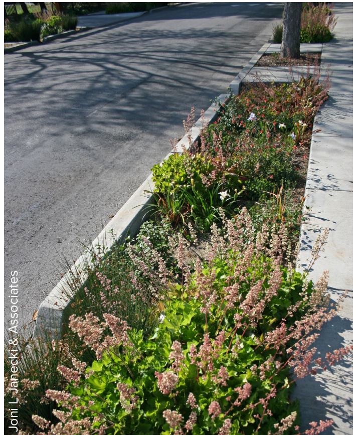
Green Street with Bioretention
