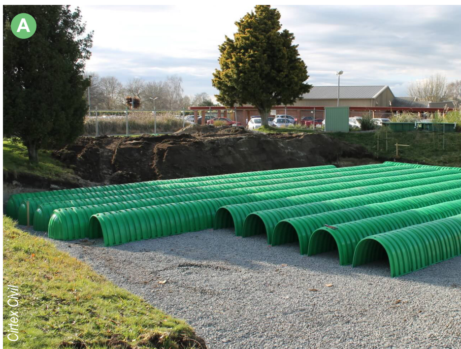
Example of Subsurface Infiltration Chambers at University of St Thomas in St Paul, MN
