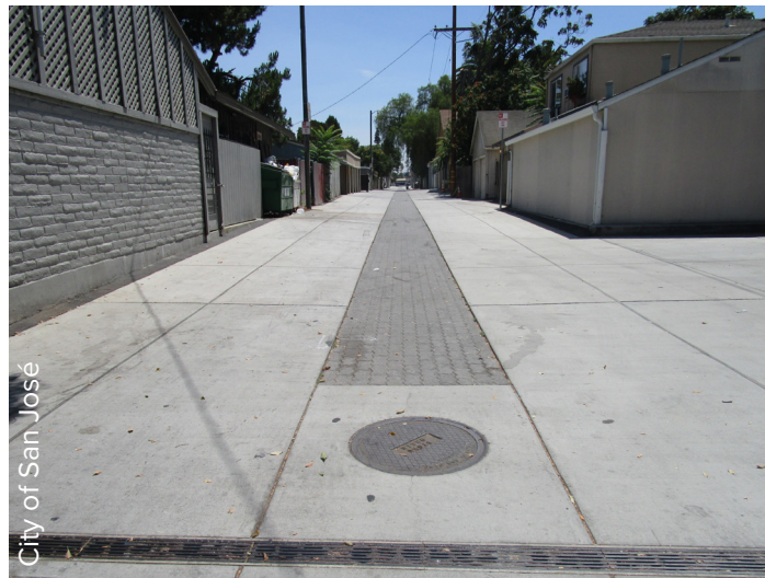
Permeable Pavement in Martha Gardens Alley Way
