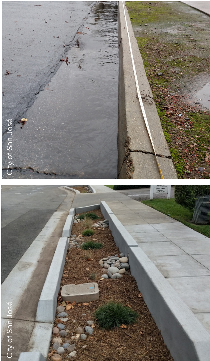
Figure 6-6. One of the Bioretention Areas Along Park Ave – Before and After
