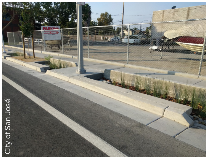
Linear Bioretention Facilities on Autumn Parkway
