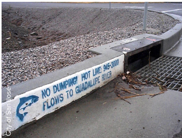
Storm Drain Draining to Guadalupe River
