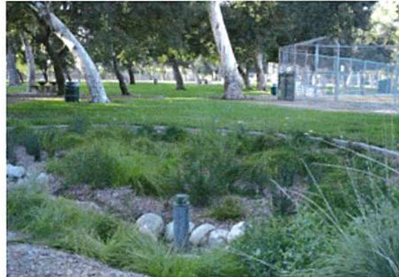
Figure 4. Sun Valley Park vegetated swales in Los Angeles County, California. (Source: U.S. EPA)
